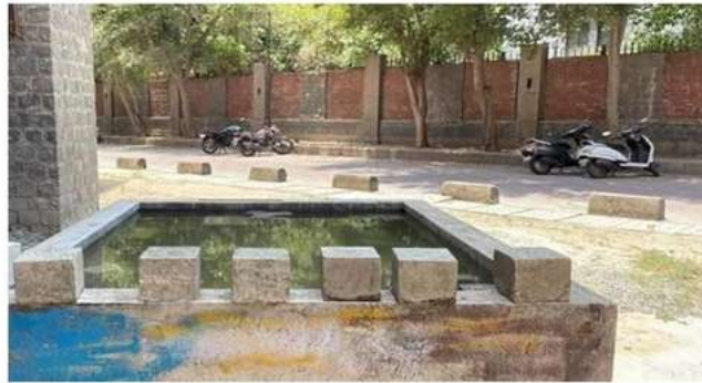
Fig. 5: Curing of Concrete
